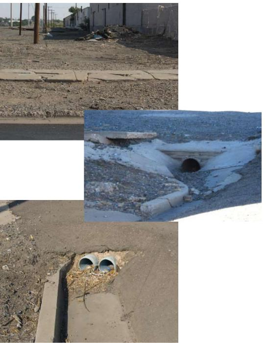
Deteriorated sidewalk and inadequate storm drainage systems are evident
